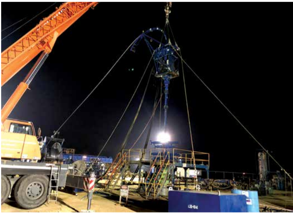
This coiled tubing operation at a Khuff gas well site on the Khursaniyah onshore field is a first for Saudi Aramco's Northern Area Oil Operations (NAOO). Through training and on-site participation of the organization's young engineers and operators in the gas well's rigless completion activities, NAOO now has a competent gas well completion team in place that is ready for future projects.
