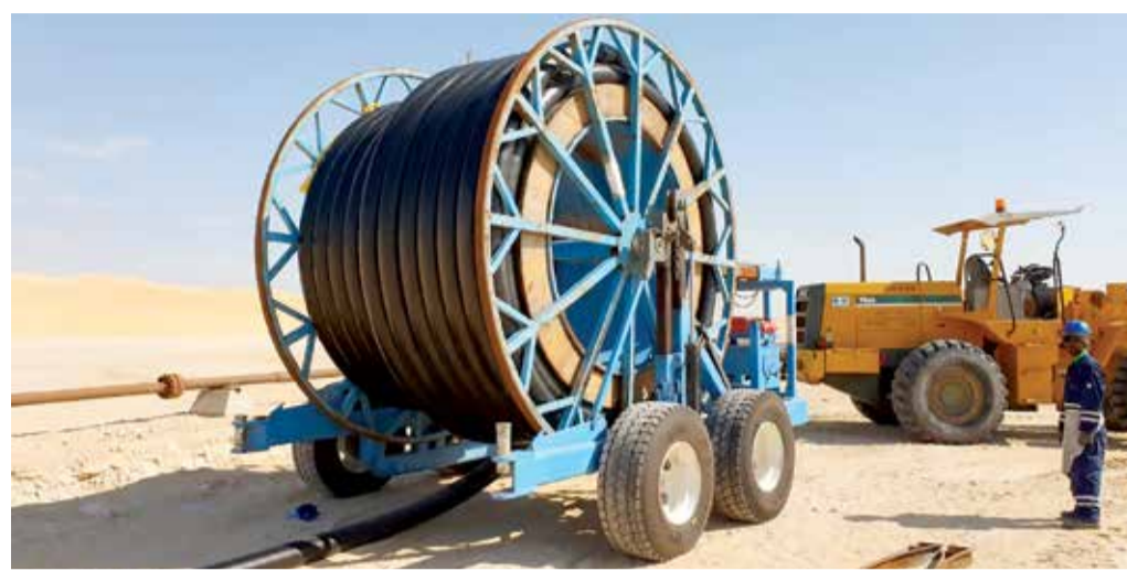
Steel-reinforced thermoplastic pipe (s-RTP), shown here being deployed in the Hawiyah area, provides a more reliable and proven way to transport crude oil under high-pressure, high temperature conditions.
